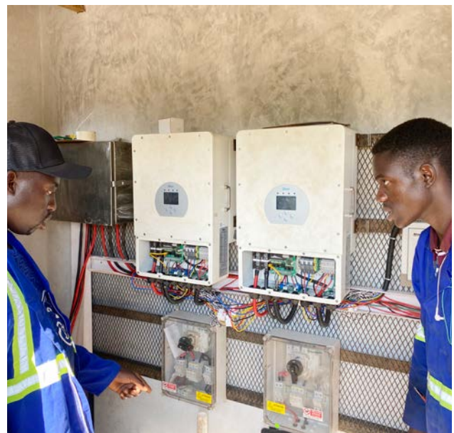
■ Image 02. Solar installation 2 installed inverters. Kuwala_2023.
