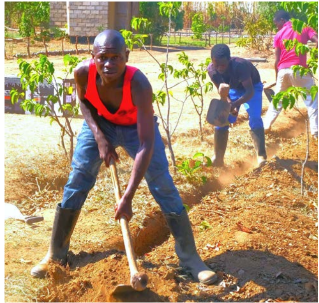
■ Digging trenches for solar cables. Kuwala_2023.
