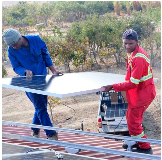
■ Roof-top solar panel installation. Kuwala_2023.
