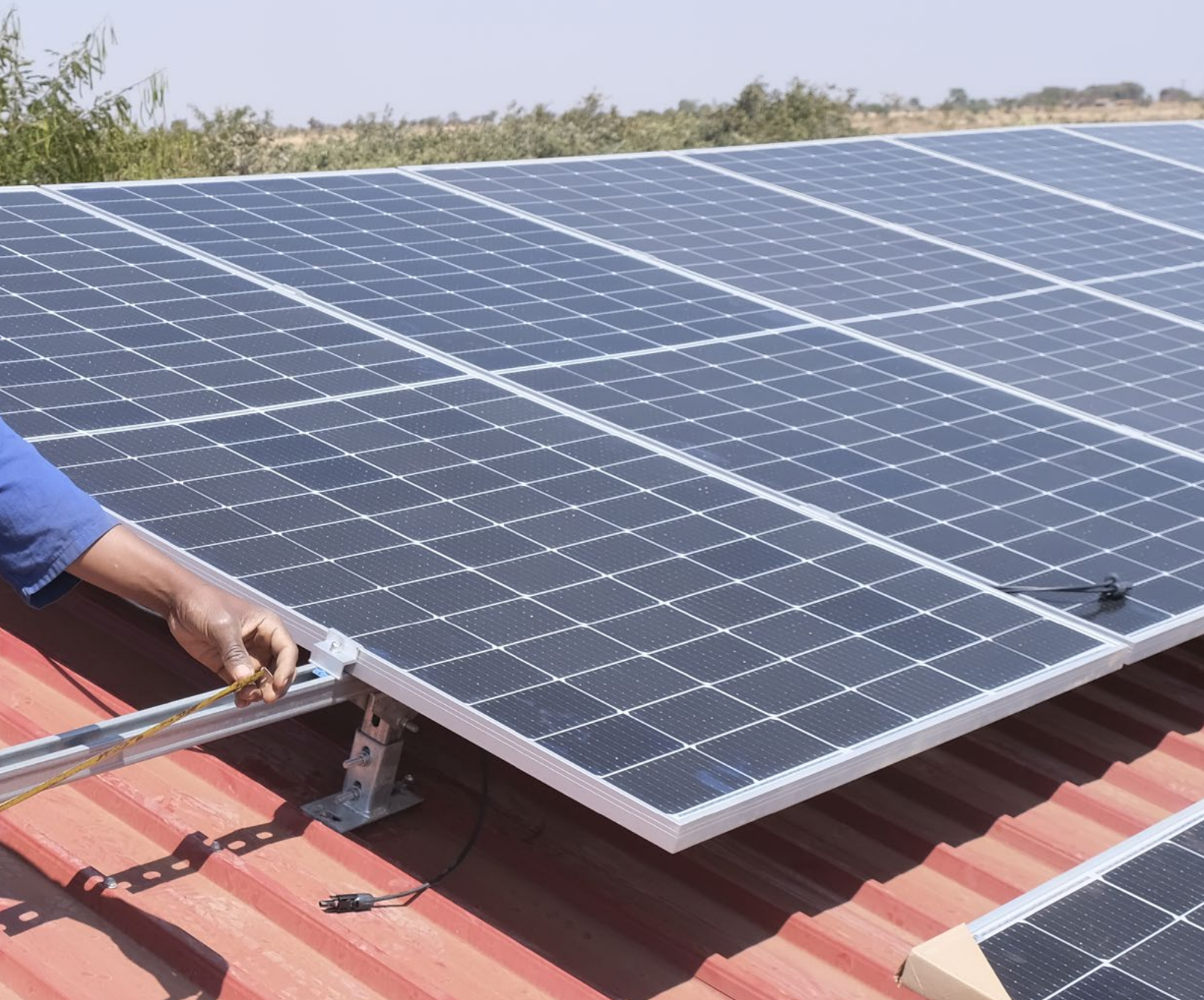
■ Securing the solar panels to the racking system on the roof. Kuwala_2023.
