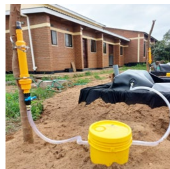
■ Biogas fields, inset photo shows gas filter and breather. Kuwala_2023.
