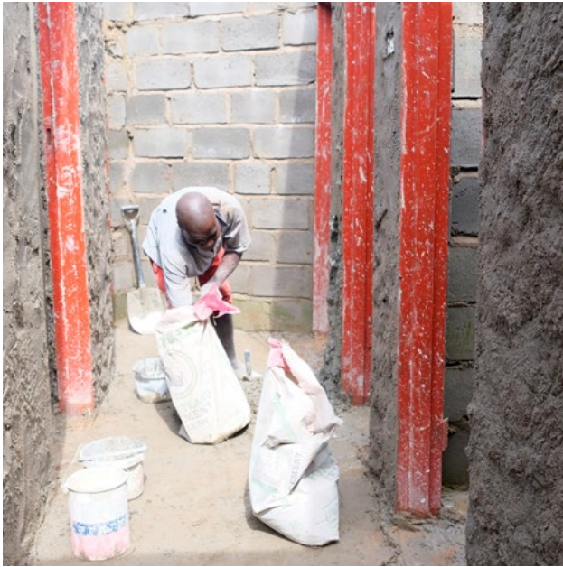
■ Plastering in progress in 2nd duplex. Kuwala_2023.
