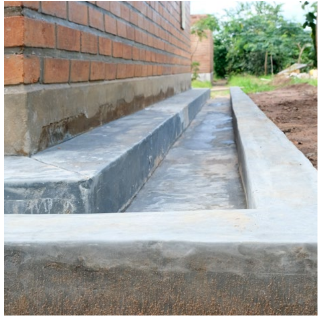
■ Water drainage constructed at 1st duplex. Kuwala_2023.
