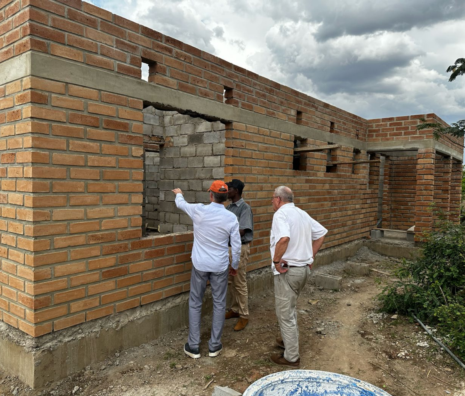
■ Commercial grade construction quality showing the staff duplex No.2 under construction with the interior and exterior walls up to the roof level. Kuwala_2022.
