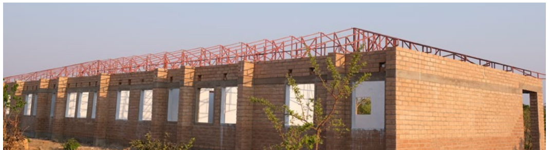
■ Second classblock is wearing a hat of metal trusses for the roof. Kuwala_2022.
