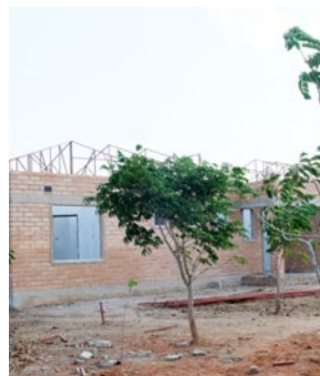
■ 1st image: 1st Duplex staff house roof trusses, 2nd image: 2nd Duplex staff house foundation. Kuwala_2022.
