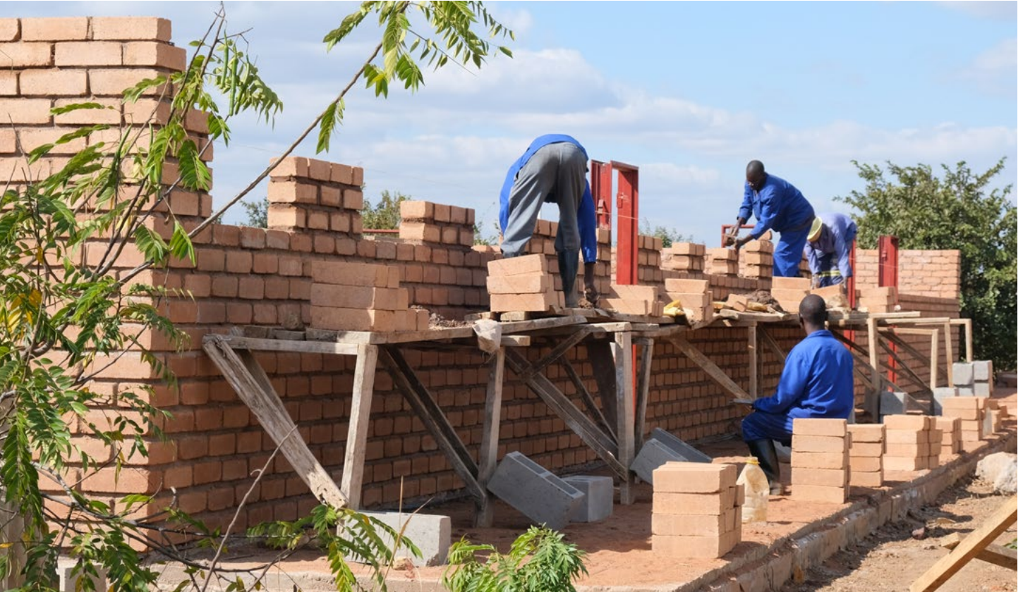
■ Second classroom block walls going up, front exterior view. Kuwala_2022.
