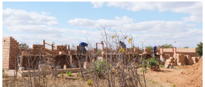
■ Second classroom block construction site, Kuwala_2022.
