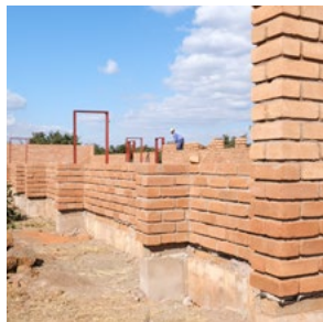
■ Second classroom block, exterior wall backside, Kuwala_2022.
