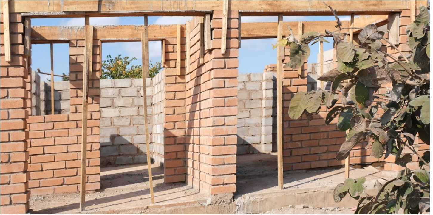
■ First staff duplex, interior showing header beams being leveled. Kuwala_2022.
