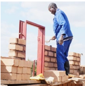
■ Second classroom block, brick and mortar install around doorway, Kuwala_2022.
