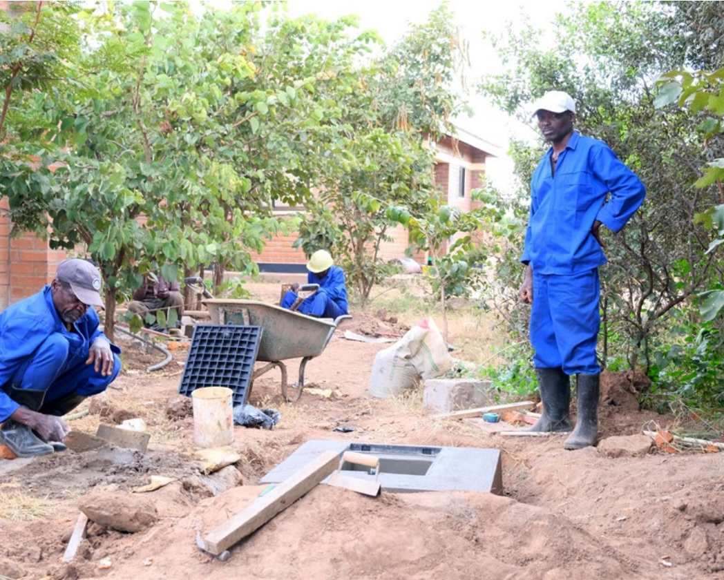
■ Men working on the staff house making a manhole, Kuwala_2022.
