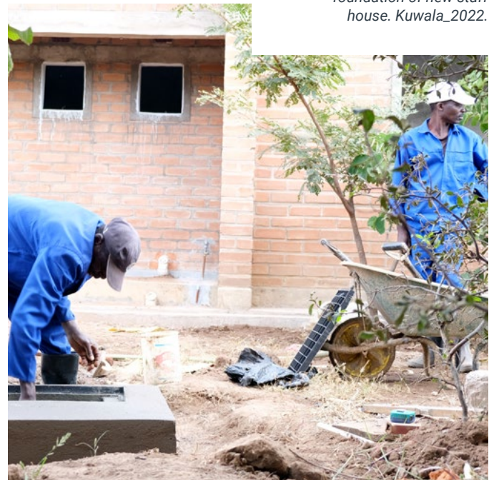
■ Making a manhole cover on staff house, Kuwala_2022.
