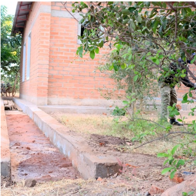
■ Water drainage construction on staff-house, Kuwala_2022.
