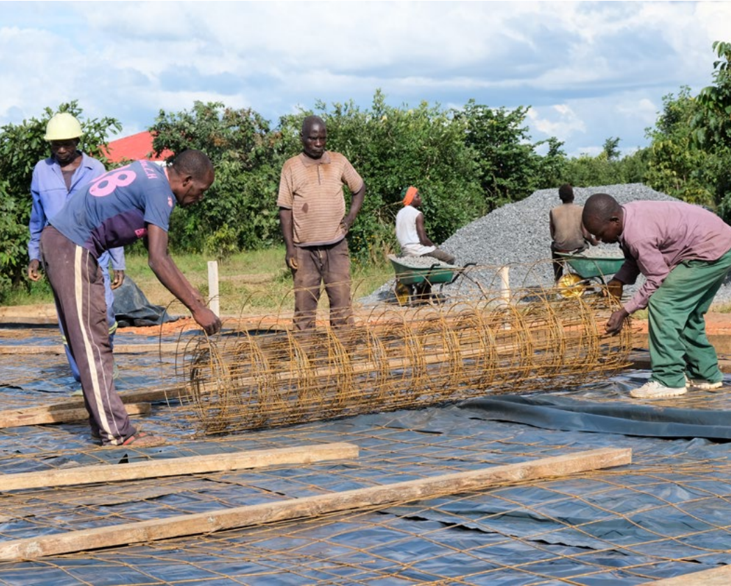
■ Top LH floor and foundation has started on the second classroom block, Workers are laying reinforcing steel for the poured concrete floor: Top RH: Old kitchen used to store onions: we have funding secured for a trades workshop and are about to start renovations.. RH middle: workers installing drainage system for St. Peter's Assembly Hall. RH bottom: electric hot water installation on second staff house. Kuwala_2022.
