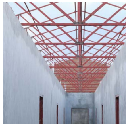
Interior of the second hostel. Steel for the roof instead of wood for the trusses are used. Kuwala_2021
